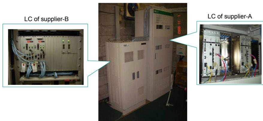
Fig 4: Overview of the two prototype of the LC
