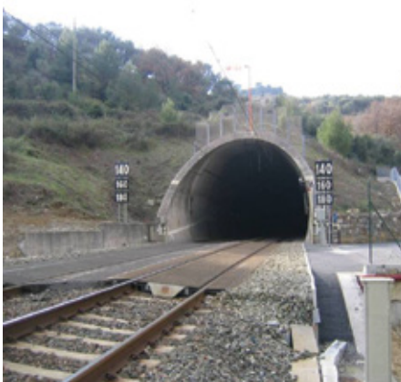
Figure 2 – Example of fence above the entrance
