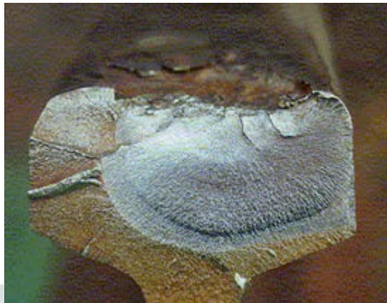
Rail Squats are a form of Rolling Contact Fatigue
