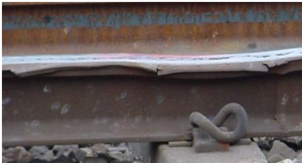
Low Rail Rolling Contact Fatigue & deformation
