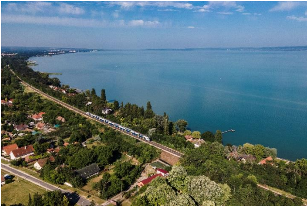
Several railway lines serve tourist needs, including to Lake Balaton. Source: MAV-START
