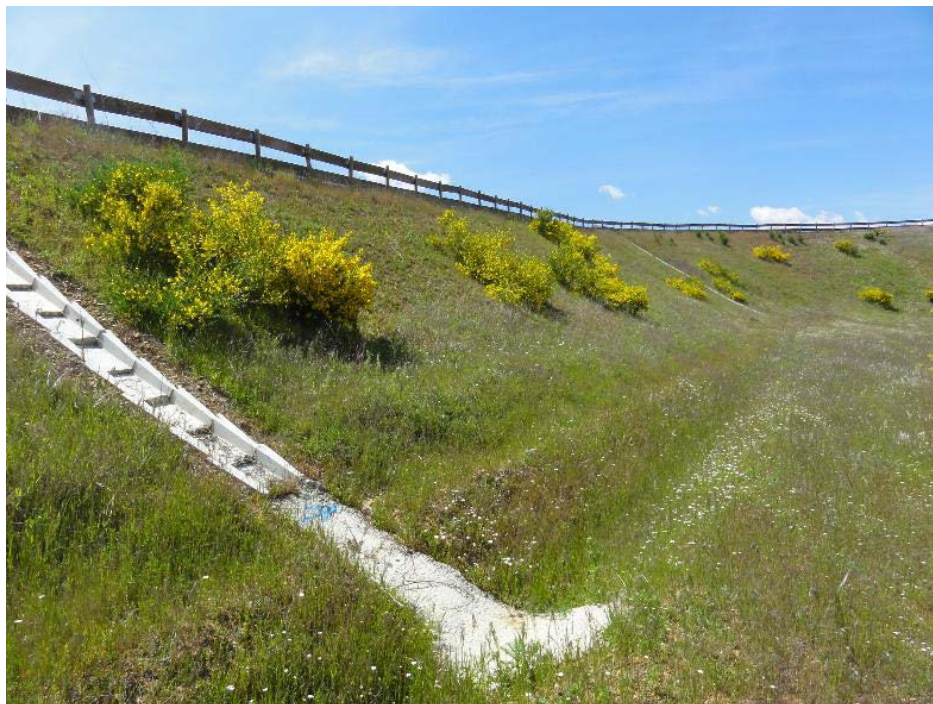
Figure 4: Embankment covered with grassland (ADIF, n.d.)
