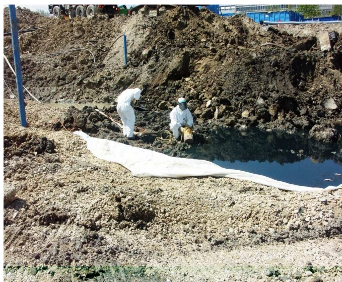
Onsite remediation, oilphase removal
