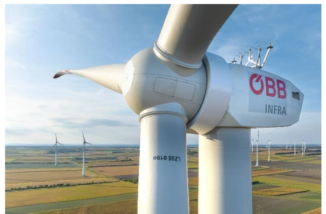
Wind turbine operated by ÖBB Infra. Source: ÖBB
