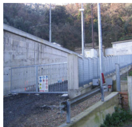
Figure 3 – Shafts: example of a fence around shaft entrance
