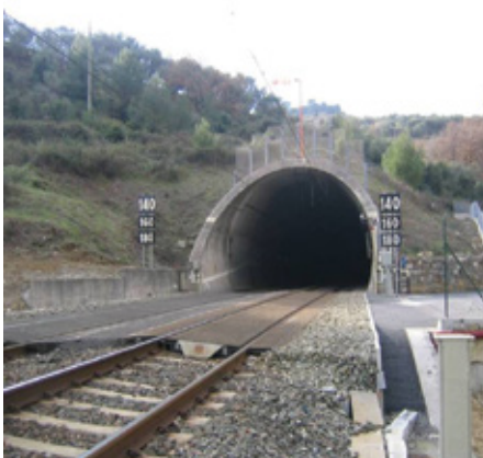
Figure 2 – Example of fence above the entrance
