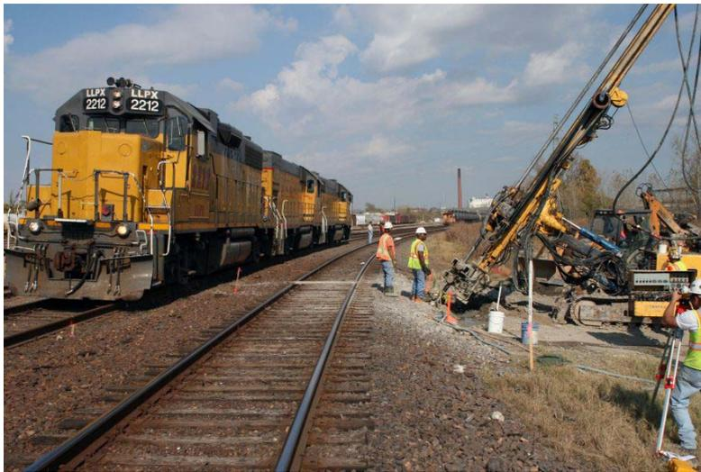
**Graph 30. Jet grouting of piles/columns under an existing railway to compensate for very soft ground. © Hayward Baker, Inc., photographer: Jeffrey Hill.**
