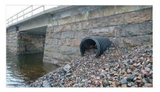
Figure 15: Pipes and ducts to facilitate movement of medium-sized mammals under Swedish railways, © Trafikverket
