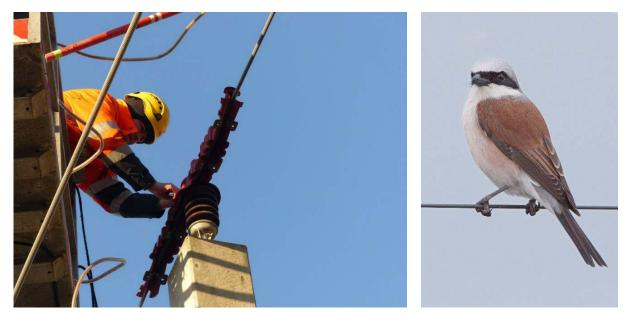
Figure 28: Measures to reduce the number of these short circuits - application of a guarddevice in front of the insulator and a bird protection cap on top of the catenary pol (left) Lanius collurio (right) © ÖBB - Infra
