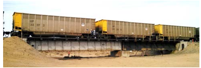
Figure 6. Photograph of a steel bridge span at FAST.
