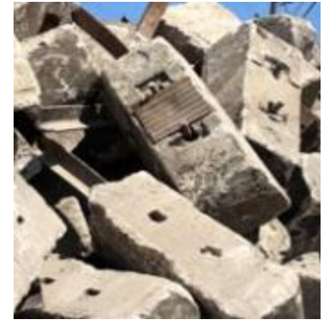
Figure 18 : used pads stuck to concrete sleeper
