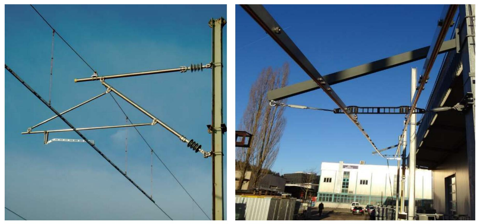
Profile to be added on an existing catenary to be contact wire and pantograph Reinforced OCL
