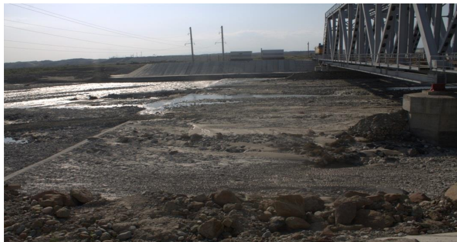
River bank protection work
