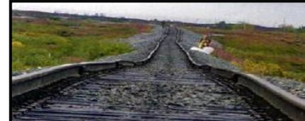
Track deformation on the Kharp – Labytnangi line caused by cryogenic processes
