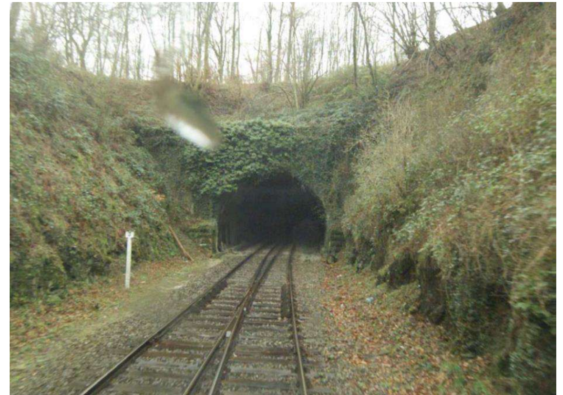
L132 tunnel with interlaced tracks (and many more obstacles and difficulties)!!
