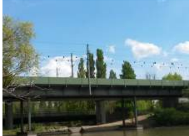
Discs to make overhead line visible for water fowl
