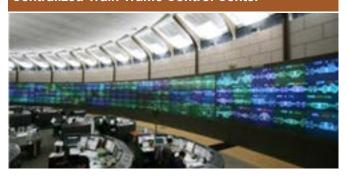
KORAIL operates and monitors more than 89%, out of about 4,200 km the total service length, by Centralized Traffic Control Center. The nationwide trains, which are KTX, conventional and freight train and subway in metropolitan area, are under control of the center. This center is essential for the safe rail service with various advanced technology of signal and IT, and knowhow from all sectors in railway. It also is control and manage incidents for quick and safe restorage in railway lines.
