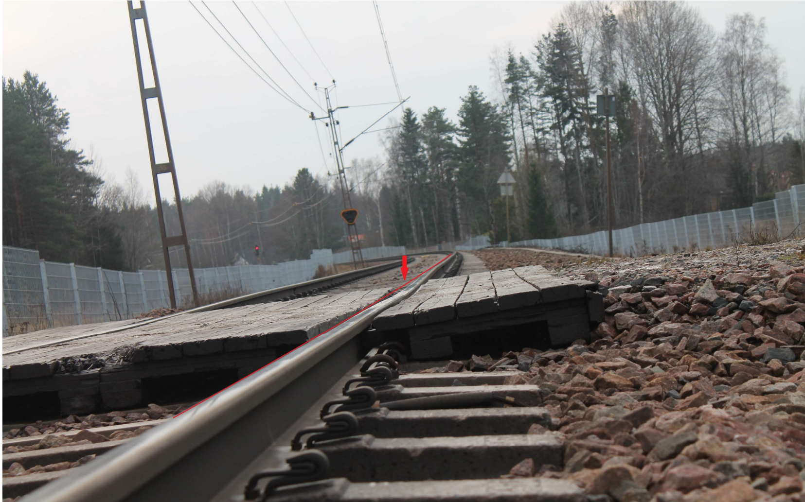
EXAMPLE OF AN ALARM, UNDERMINATION CAN COME SUDDEN AND CAUSE ACCIDENTS
