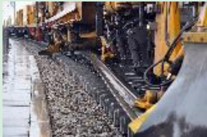
SUZ 500 Track (Re)Laying
