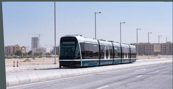
Lusail tramway project in Qatar © ALSTOM
