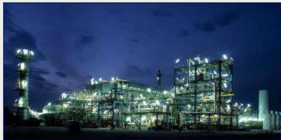
Air Liquide, Port Jerome (SMR +CCS)
