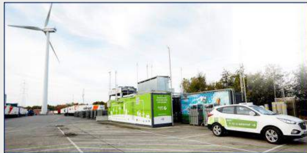
Colruyt Group, Halle (Electrolysis +RE)
