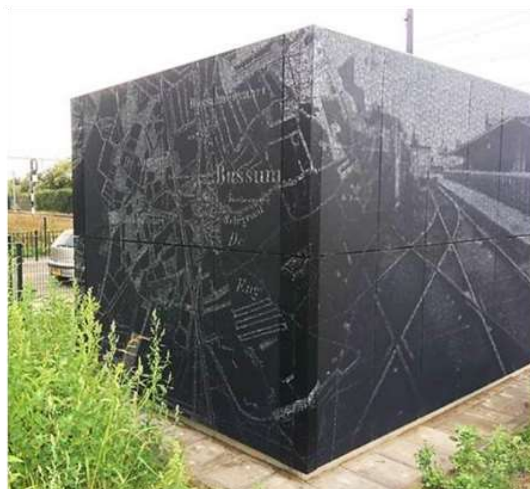
Energy wall (tech. build.)
