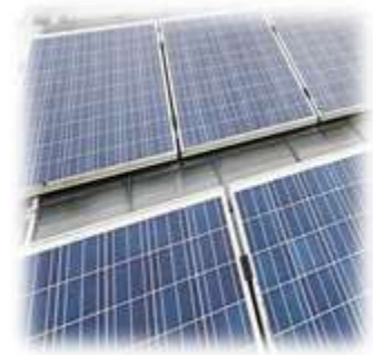
Solar Panel installation
