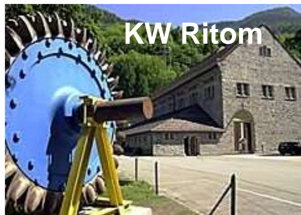
60 MW (new 16.7Hz Turbine & Generator)
