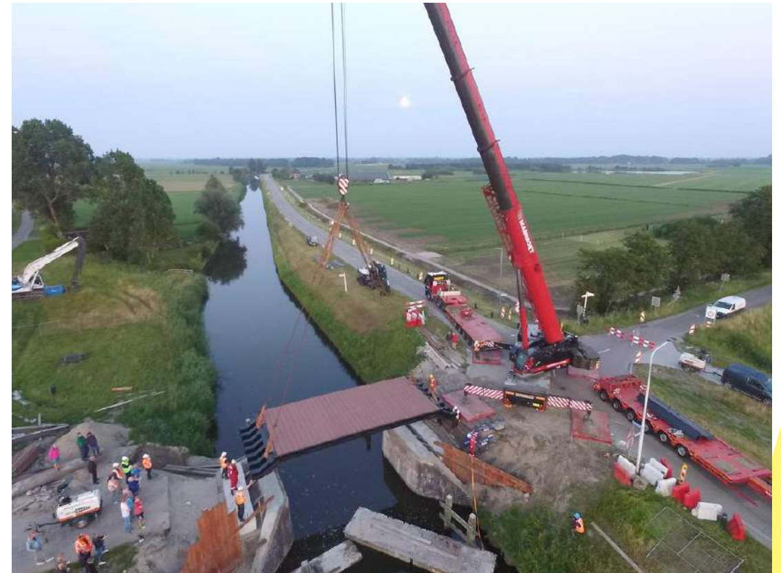
Installation of the bridge deck of re-used composite
