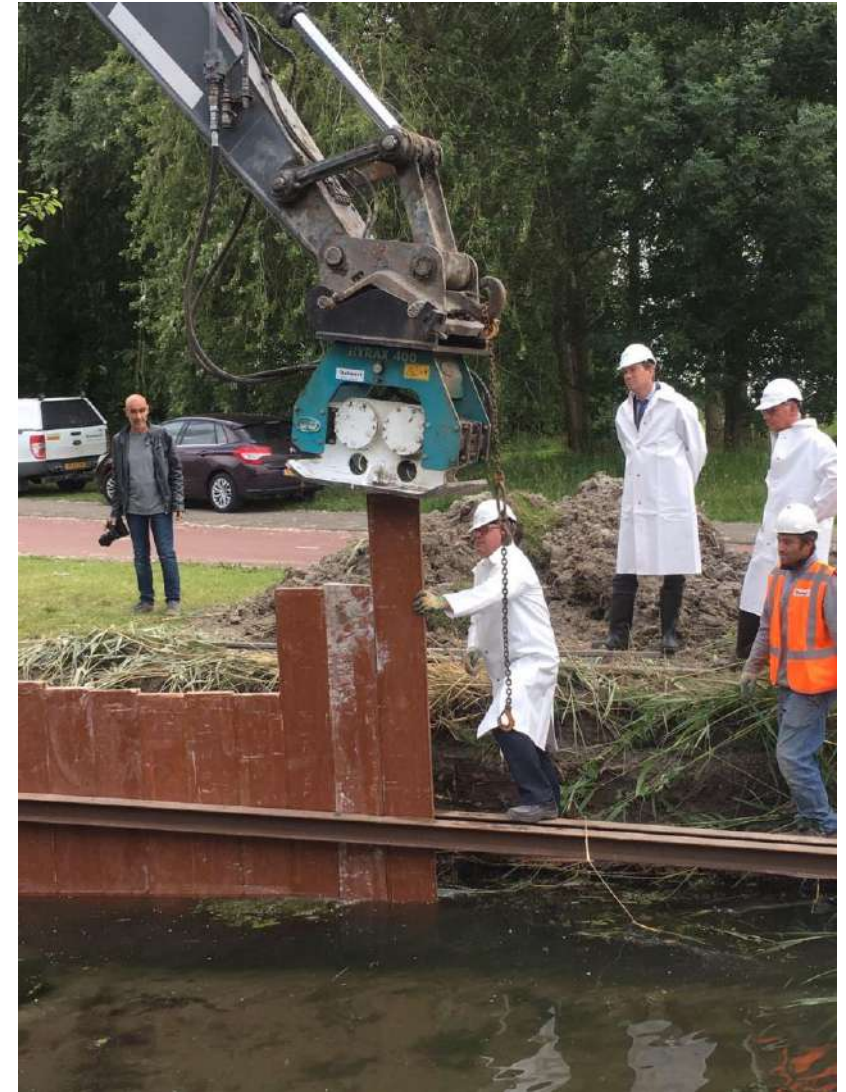
Installation of retaining wall
