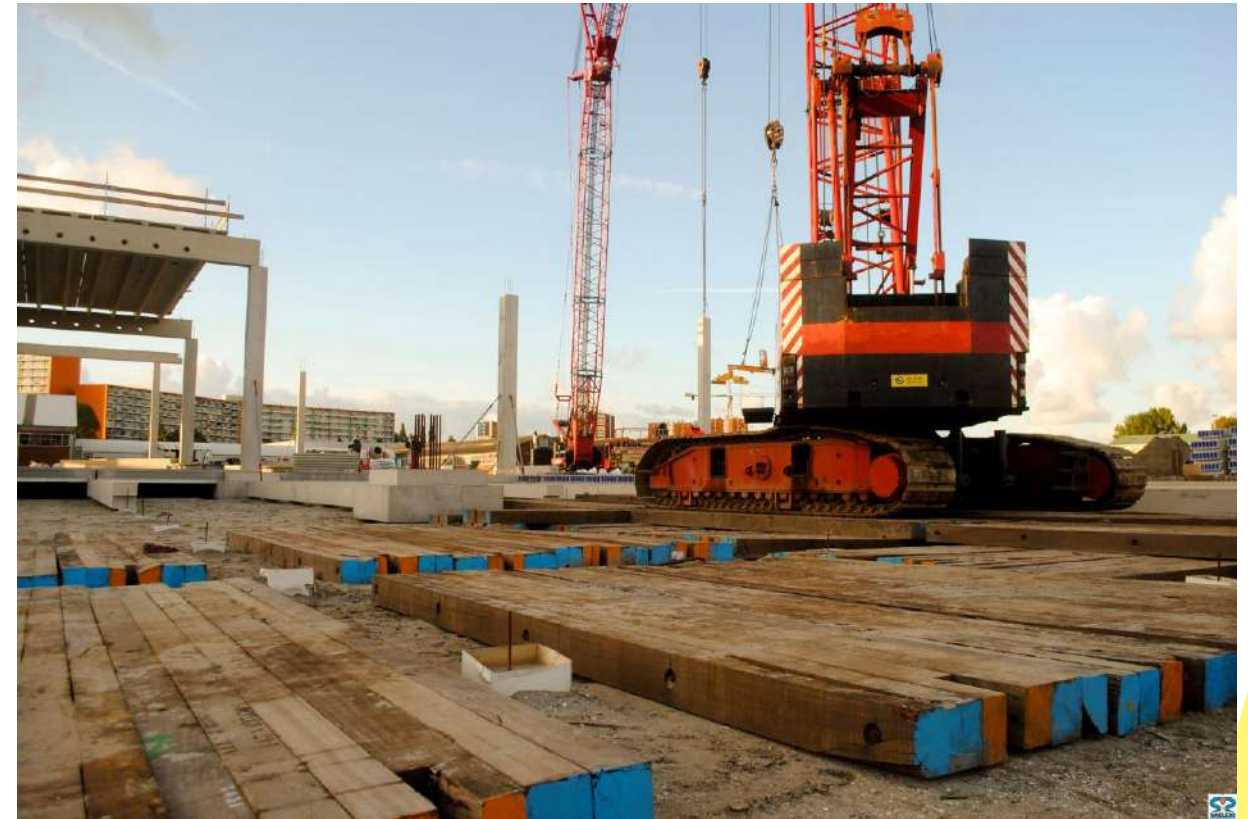
Crane mats of Welex at a building site
