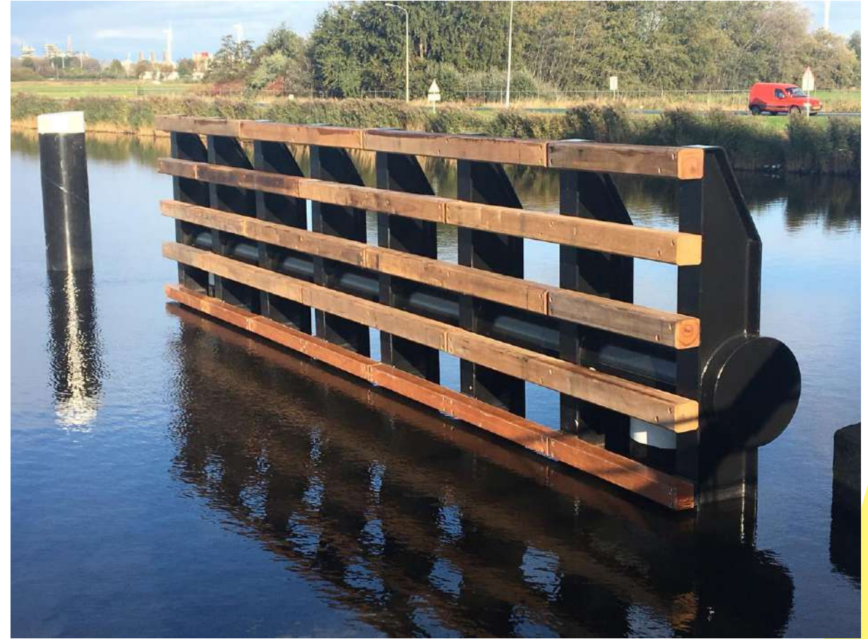
Guiding structure near Heemkes bridge
