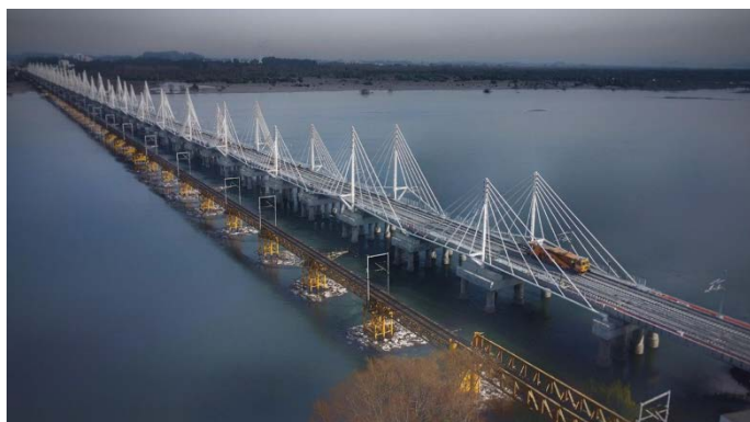
Figure 16: Train passing over the new Biobío Railway Bridge in Concepción, Chile. Source: EFE, 2025
