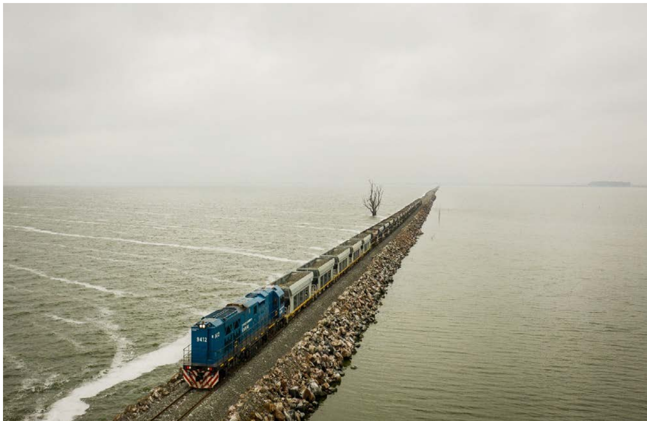
Figure 10: Belgrano Cargas train passing over a stone embankment on the La Picasa lagoon. Source: FASE, 2025
